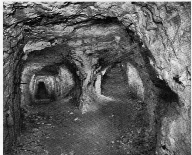
Junction with Cannon Road car park branch entrance tunnel to the right. A short distance along the left tunnel there is a T-junction with Ellington Park entrances to the right and Hospital and West Cliff Harbour entrances to the left. This part of the tunnel network now carries a sewer pipe with no access possible.
